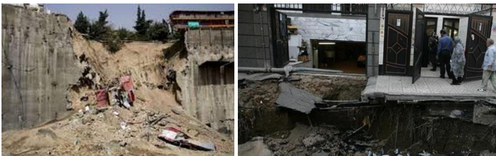
Fig 12. Examples of collapse of such excavations taken from lecture by Prof. Fakher of Teheran University (Fakher, 2013)
